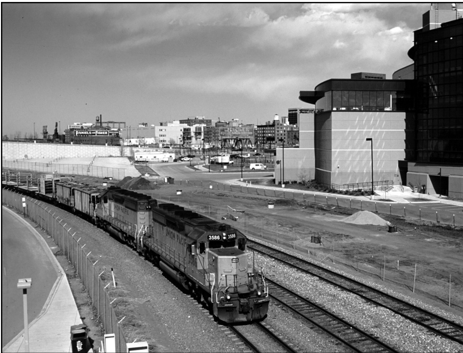
Union Pacific empty rail train passes the Pepsi Center where the new Regional Transportation District line is under construction. UP SD40-2 3586 was moving south on April 19, 2001. Construction to the right will be an RTD station for the Pepsi Center and Six Flags Elitch Gardens. – Photo © Chip.
